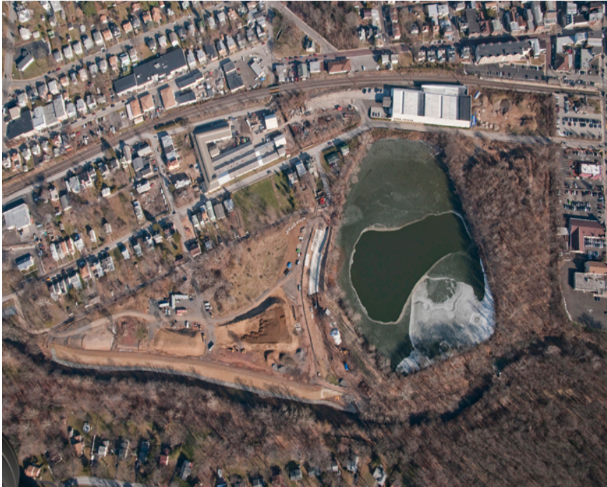
BoRit Superfund Site Aerial View
